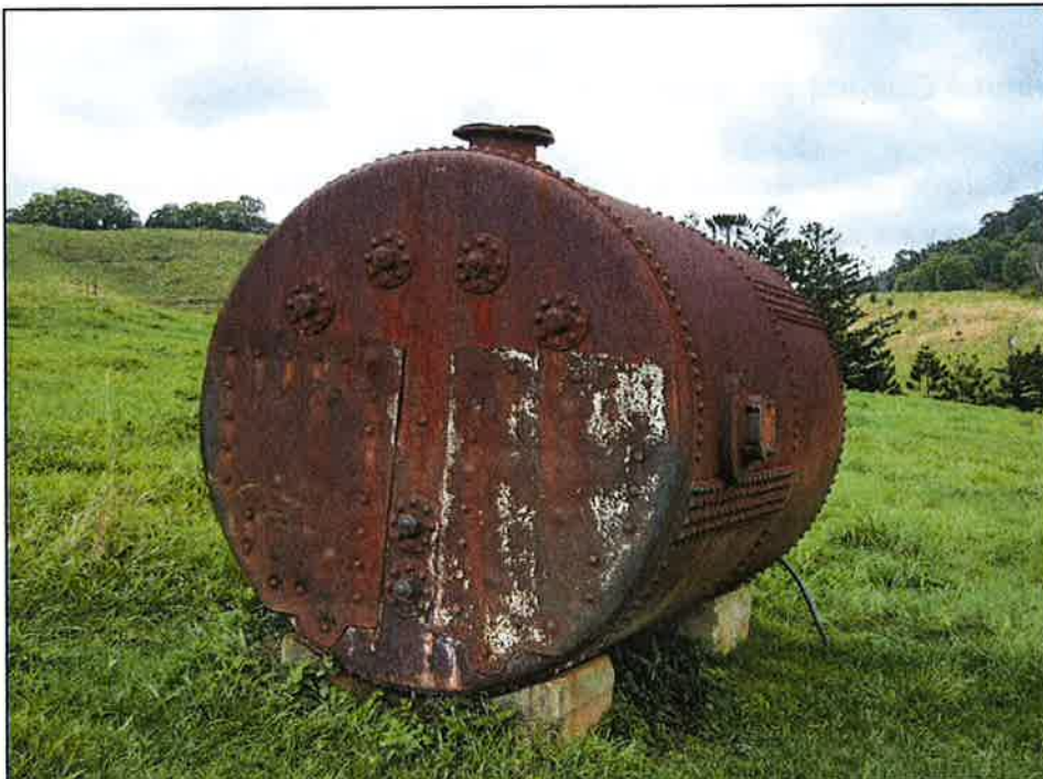
Figure 22: View of Steam Boiler
